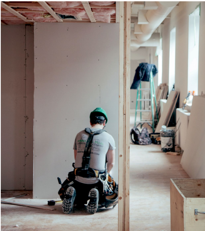
Insulation, a key energy-efficiency measure, gets installed in Montreal, Canada.
